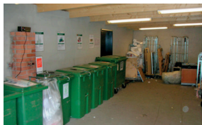
AirMaid® i affaldsrum
